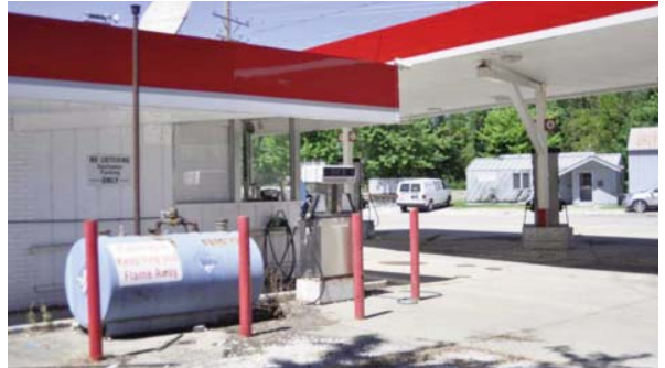
Leaking tanks at gas station in Highland, Illinois.
