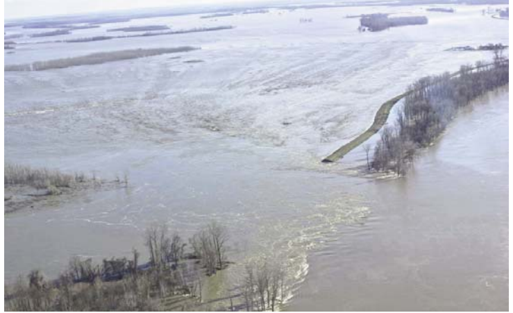
A breach in the Len Small Levee last year in Alexander County flooded thousands of acres in and around Horseshoe Lake State Fish and Wildlife Area. The flooding created a nightmare scenario for wildlife as well as residents of the area. Photo provided by the Illinois Department of Natural Resources.
