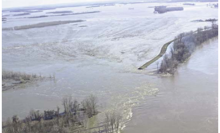
A breach in the Len Small Levee last year in Alexander County flooded thousands of acres in and around Horseshoe Lake State Fish and Wildlife Area. The flooding created a nightmare scenario for wildlife as well as residents of the area. Photo provided by the Illinois Department of Natural Resources.
